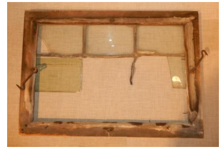
An original window, with lead between the glass panes, survived in the Sisters’ House. This is the type of window Michael Miller made, and in 1762 he made windows for the Sisters. Did he make this one?
